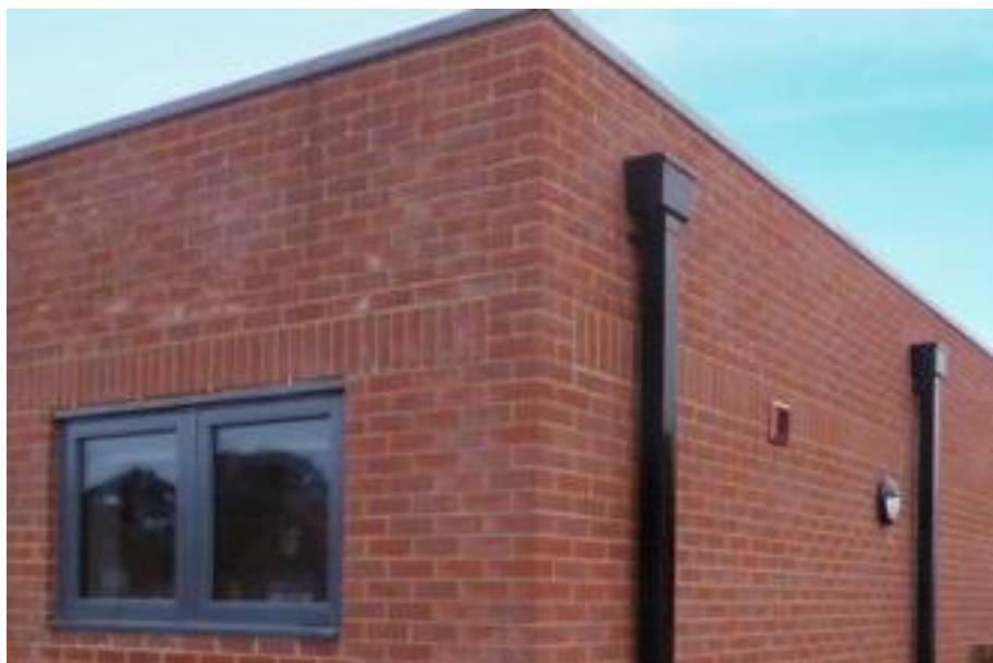
SEN & Library: PPC Aluminium windows, coping cappings and rainwater goods
