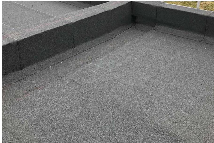
SEN & Library: Bituminous felt flat roof
