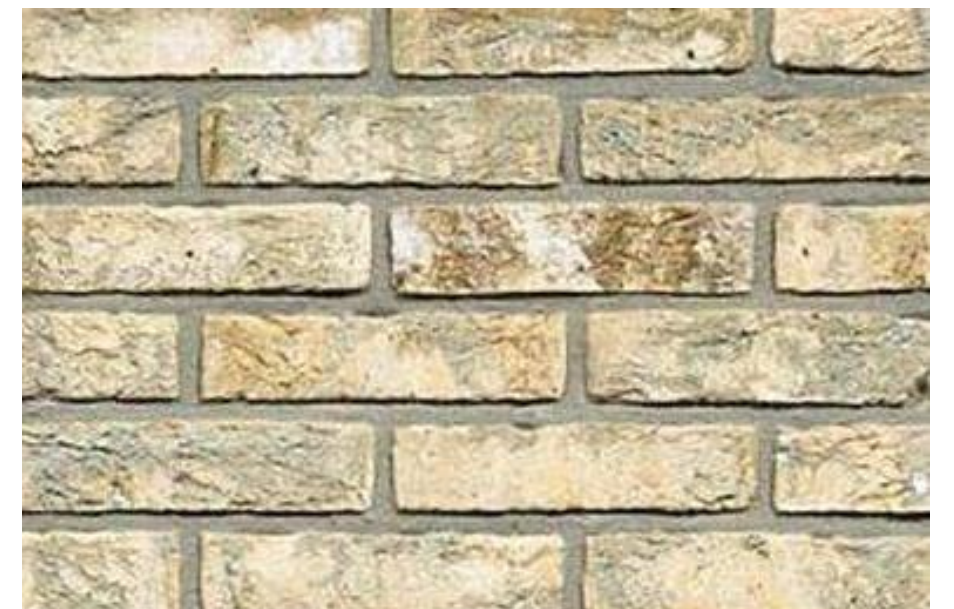
SEN Extension: Buff stock brick to match 2013 expansion
