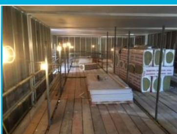
The above pictures show the cladding and insulation works being undertaken to the inside of the building. This will be followed by screeding of the floors and first and second fixings for the electrical system
