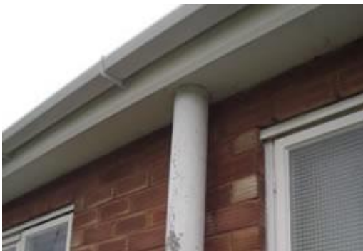
Asbestos cement drainage pipe (downpipe)
