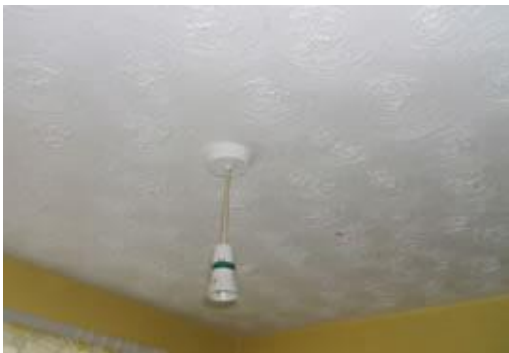
Asbestos textured coating
