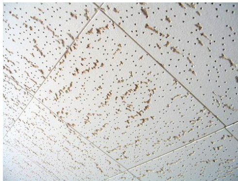
Asbestos containing ceiling tiles
