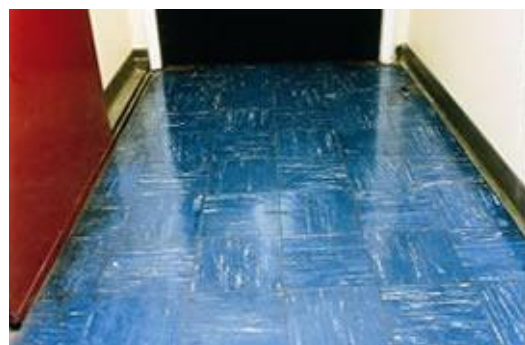
Asbestos containing floor tiles in a corridor
