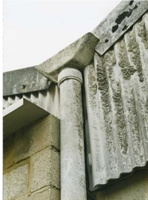
Asbestos cement downpipe, hopper and profile sheet
