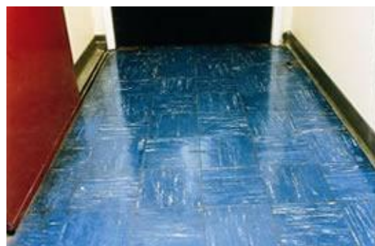
Asbestos containing floor tiles in a corridor
