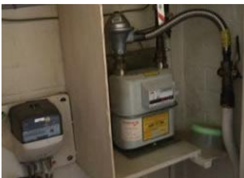
Asbestos panelling around a gas meter
