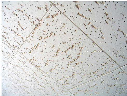
Asbestos containing ceiling tiles
