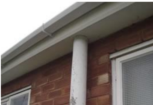
Asbestos cement drainage pipe (downpipe)
