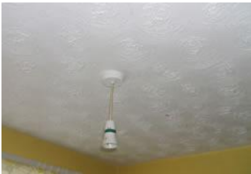
Asbestos textured coating
