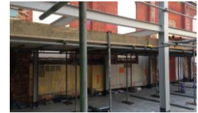
TYING INTO REAR WALL OF EXISTING CINEMA
