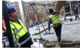
SCAFFOLDING BEING ERECTED AROUND CINEMA EXTENSION
