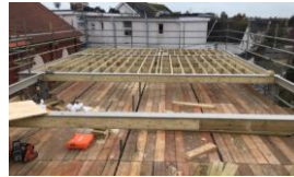
INSTALLATION OF HIGH LEVEL JOISTS
