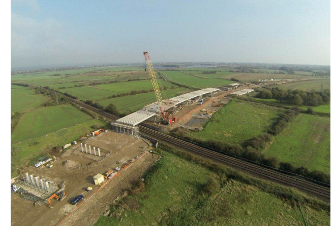
▲ A new viaduct under construction as part of the Bognor North Relief Road (BNRR)
